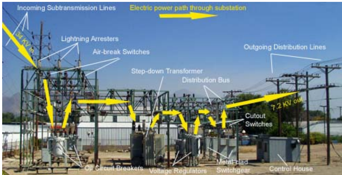
Fig. 2. Substation overview.
