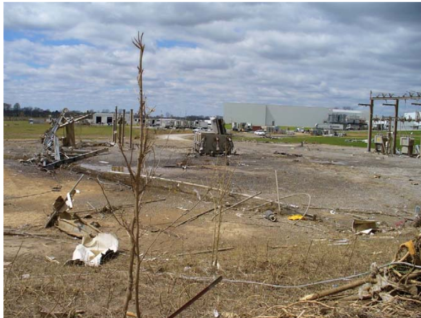
Fig. 8. Biffle Road substation tornado damage, near Dyersburg, Tennessee.
